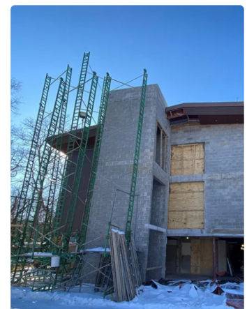
Capital High School renovation includes a new elevator.
